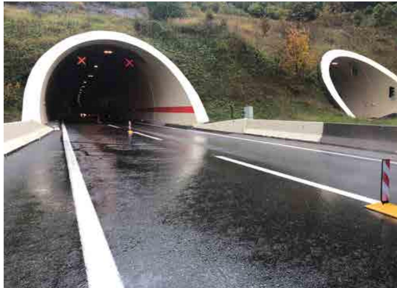
LAGE: tunnel Ledenik
